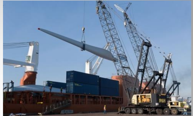
Source: Port of Houston Authority
