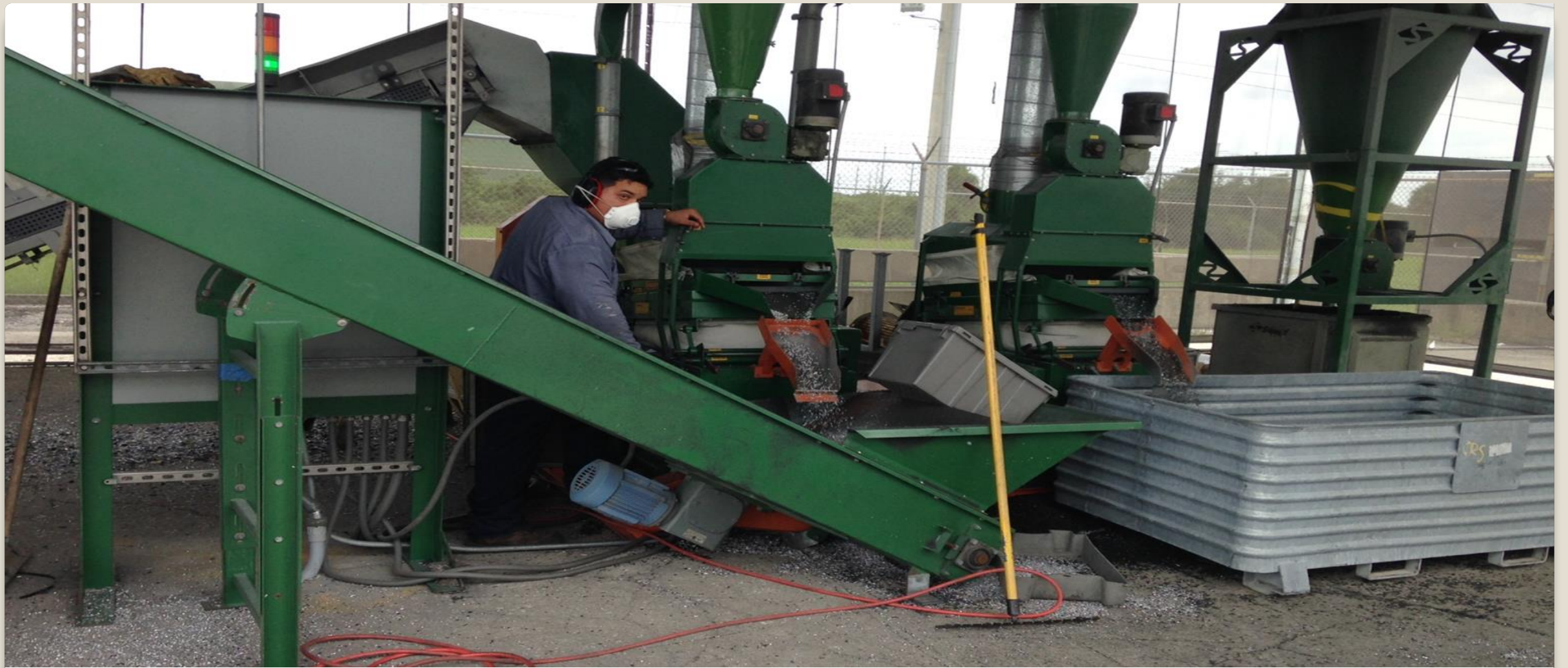
Granulator where material is further reduced and separated into aluminum and plastic jacket materials
